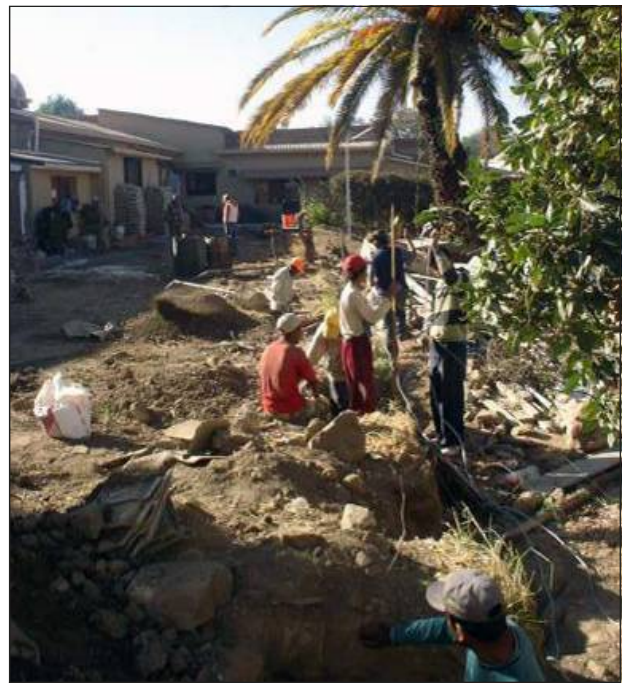
Clearing the land and getting ready to start.
