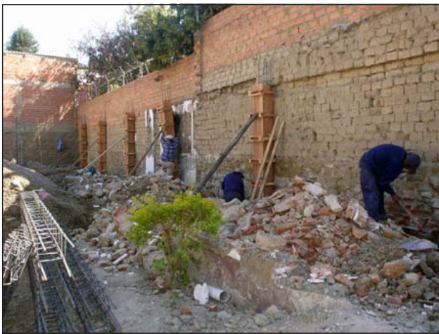
Construction is underway — July 7th!
